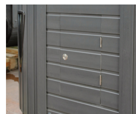
Topside is hidden behind door, only key-holder has access.
